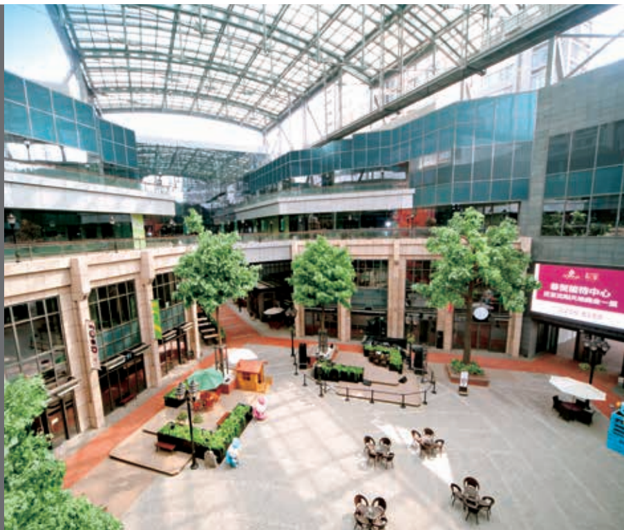
Shenyang Project Phase I
