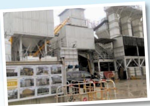
• Mobile batching plant in So Uk Estate Phase 2
