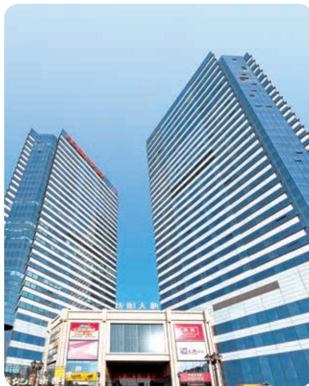
Shenyang Project Phase I
